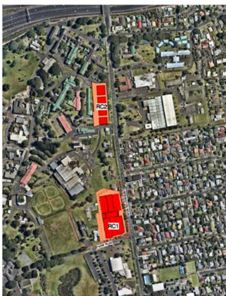
Figure 2: Consented Marutūāhu-Ockham Group RC1 and RC2 development sites fronting Carrington Road within the 10ha 'Project Maungārongo' development area.
