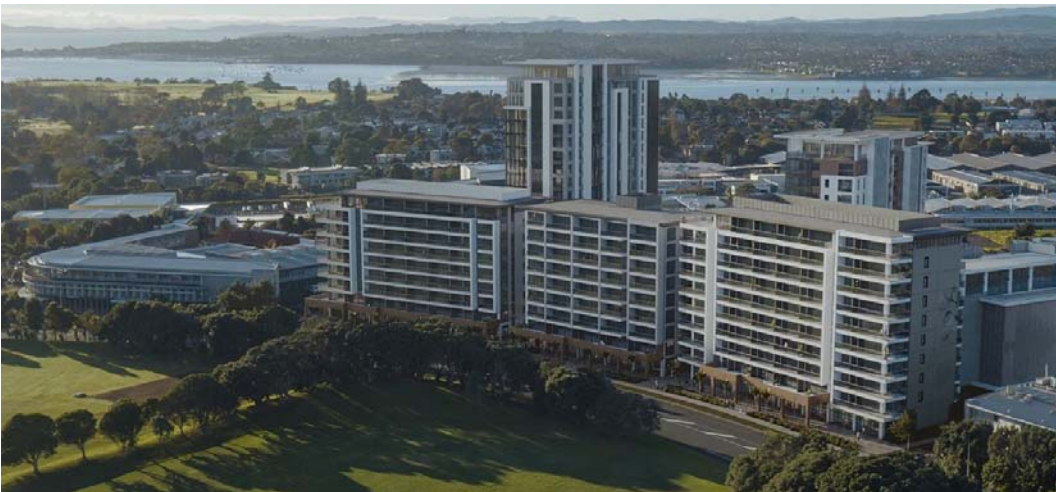
Figure 3: The Te Tauoma residential development, showing the consented Stage 1A development of three 9-10 storey apartment buildings along Morrin Road and the consented Stage 1B development of a 14 storey and an 18 storey apartment building behind.
